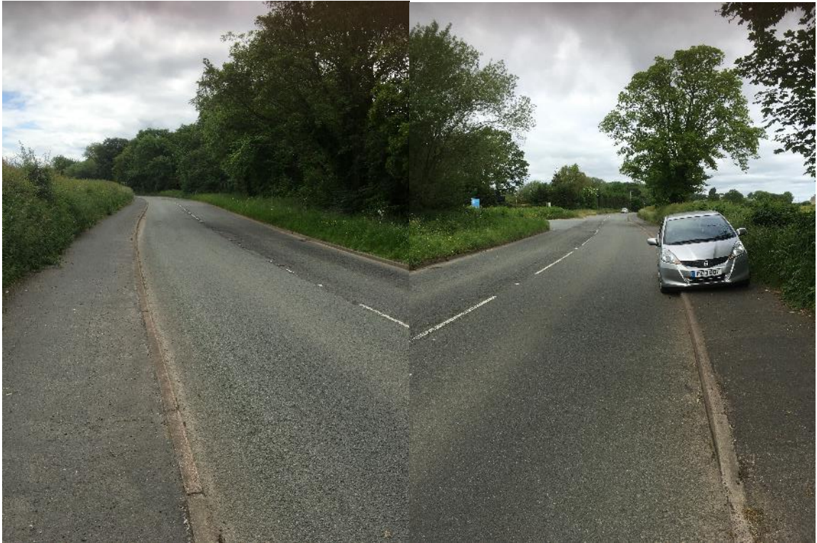
Plate 1 Visibility from Existing Agricultural Access Looking East (L) and West (R)
