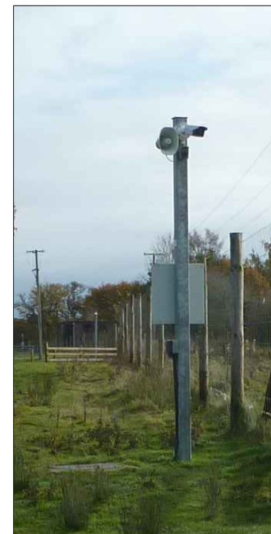
Precedent CCTV Mast
