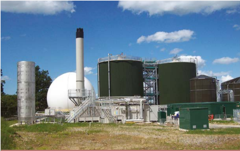
Figure 10: Five Fords Wastewater Treatment Works
